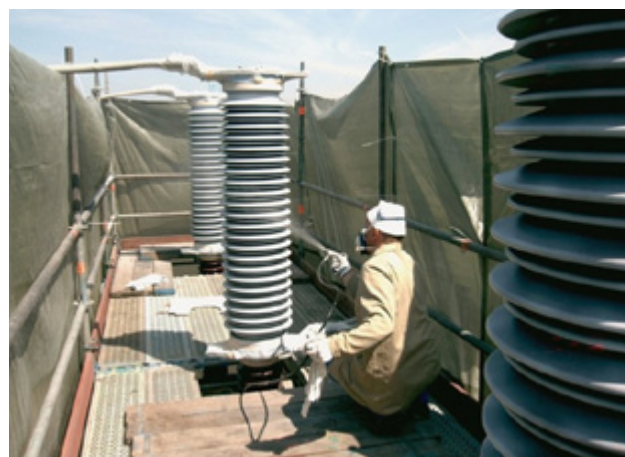
A technician applies a silicone coating to high-voltage insulators. The coating creates a hydrophobic surface that can help reduce conductive tracking and flashover risk in wet or contaminated environments. (Source: WACKER)
