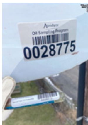
Barcode used to identify transformers. Source: Amidyne Solutions
