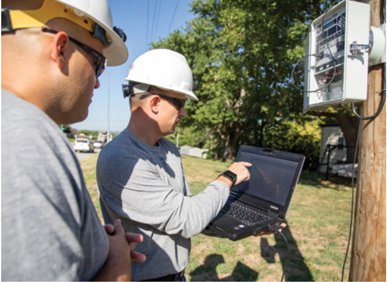
Source: Omaha Public Power District.
