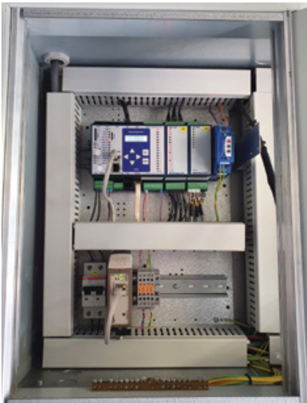
Remote telemetry units (RTUs) designed to offer flexibility and maximum security for the water, energy and industrial markets. Source: Ovarro
