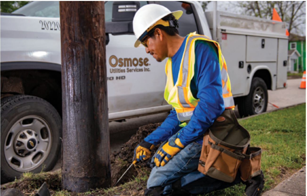
Performing a groundline inspection on a wood utility pole to detect decay. Credit: Osmose Utilities Services
