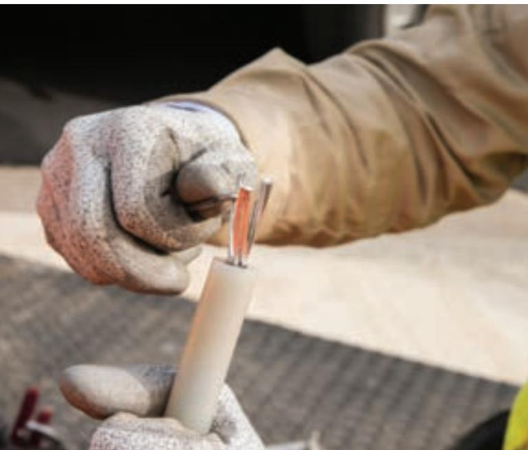
With sustained pressure rejuvenation (SPR), cables are restored to full dielectric strength in seven days, and injection can be completed in a single day. The steps are as follows:
