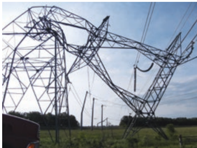
138/345kV lattice structure downed by flying debris.
