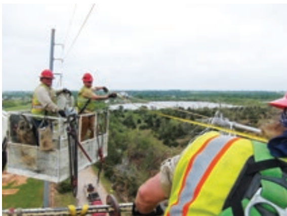
Crew measuring the damaged area of conductor in preparation for replacement.
