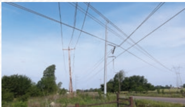
138/345kV conductors dropped on ACCC and adjacent distribution line. Note the force of the impact was great enough to snap the upper phase insulator. The impact did not appear to damage the ACCC conductor although armor rods were installed on the ACCC conductor as a precaution.
