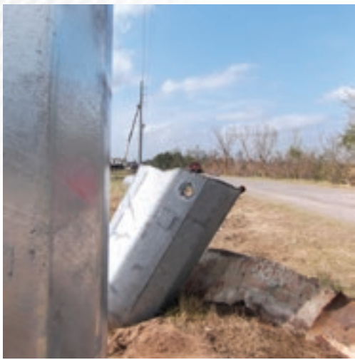
Newly installed replacement pole next to base of the damaged monopole.
