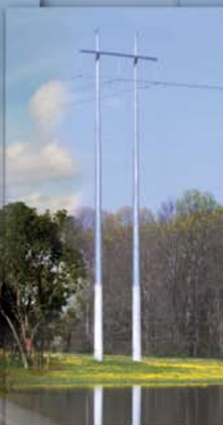
Hybrid Pole Concrete Base and Steel Upper Section
