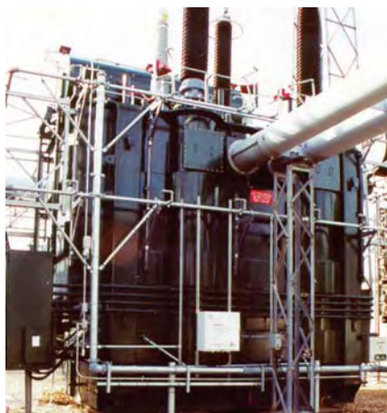
Figure 8 – Fiber optic temperature sensor on a 107MVA converter transformer
