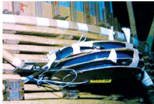
Fig. 6 Temporary spooling of fiber optic sensor
