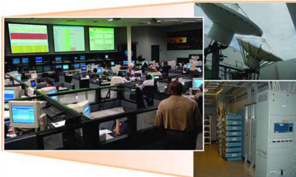
Figure 3: The USA Mobility Carrier Class 24/7 Network Operating Center and associated VSAT back-haul equipment.
