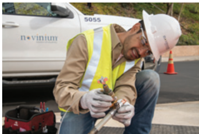
The rejuvenation fluid enters the conductor via an injection pin and injection adapter that is connected to the cable end.
