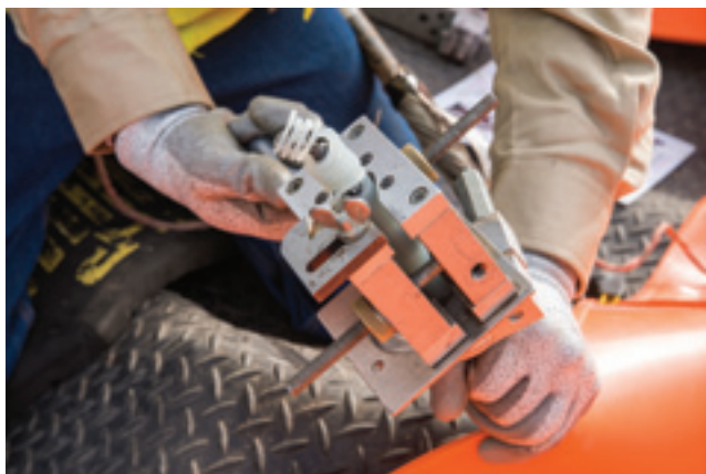
A portion of the electrical cable insulation is removed to attach an injection adapter in preparation for injection of Cablecure rejuvenation fluid.
