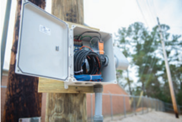
A junction box provides fiber optic communications and power for the cameras
