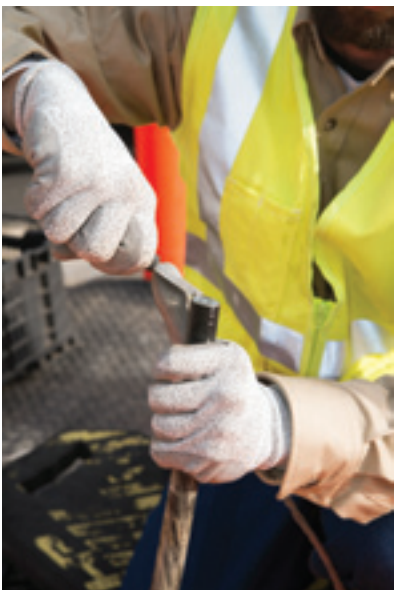
Removing cable sheath and insulation in preparation for injection.
