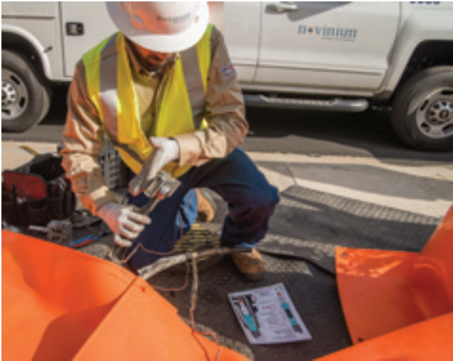
Preparation of cable for injection by removing sheath and insulation.
