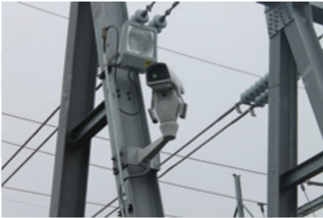
Cameras that operate in close proximity to high voltage lines require immunity to the effects of EMI.
